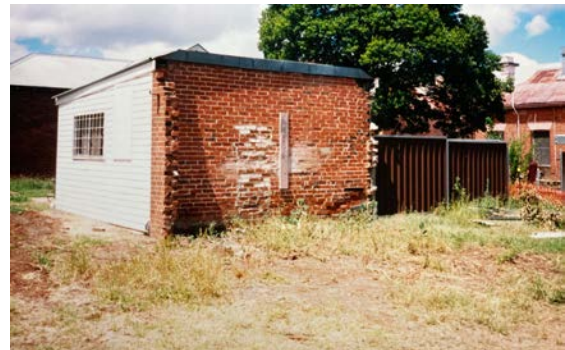
The shed at the rear of the cottage photographed in 2002 before demolition of the unstable brick wall. The attached remnants of double brick side walls were those of the former Court House Caretaker's Quarters. (Courtesy Joan Wakeford)
